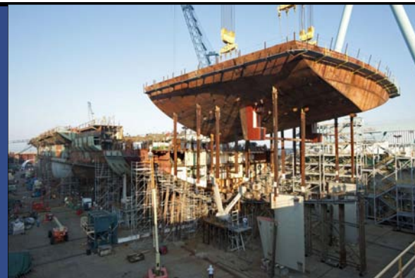
Newport News Shipbuilding completed an 825-ton superlift on the aircraft carrier Gerald R. Ford (CVN-78) on 12 September 2011. At 90 feet long, 120 feet wide and 30 feet deep, the stern section superlift was among the largest of the 162 that comprise the U.S.S. Gerald R. Ford. Photo courtesy of Newport News Shipbuilding.
