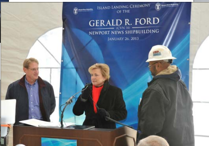
Susan Ford Bales, assisted by NNS vice president for CVN 78 construction Rolf Bartschi and veteran shipbuilder Curtis “Doc” Eley, radios the official command to crane operator David Rushing to lift and land the island of the USS Gerald R. Ford.
