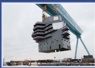
555 ton island is lowered into the flight deck of the USS Gerald R. Ford (CVN 78)
