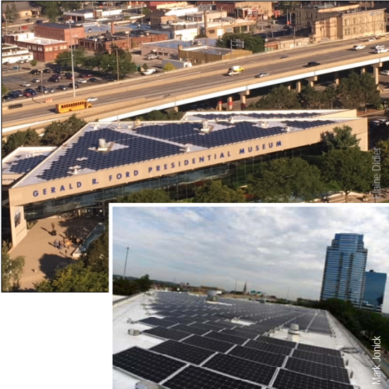
Left: An aerial photo of the museum showing the new solar panels installed on the roof. Inset photo shows the solar panel detail.
